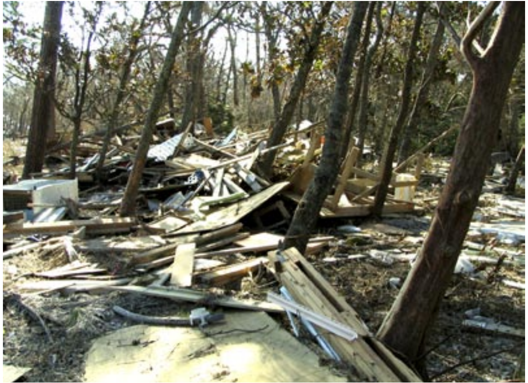
A debris field deposited by Hurricane Ivan lies outside park headquarters at Gulf Islands National Seashore. NPS PHOTO
