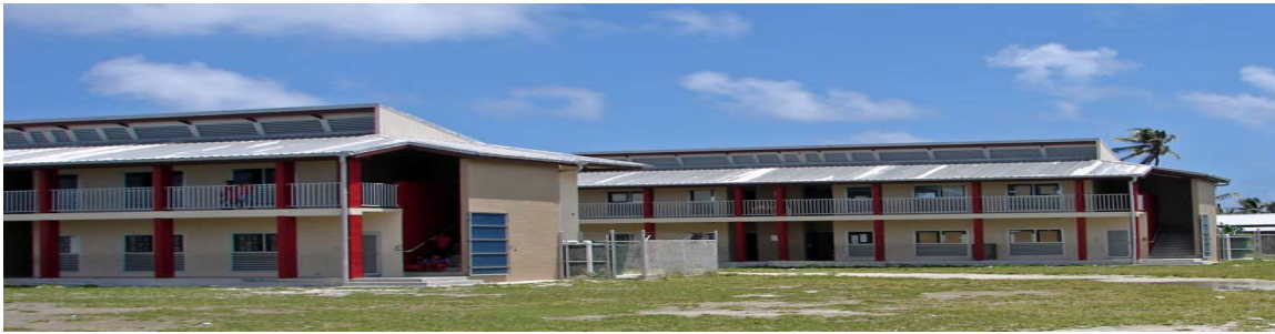
Sixty-two classrooms were completed in the Republic of the Marshall Islands this fiscal year.
