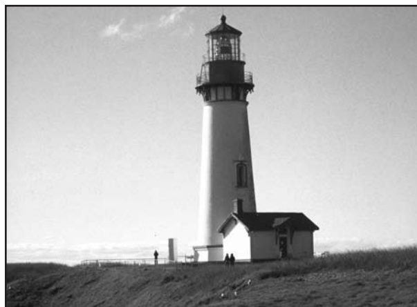
The historic Yaquina Head Lighthouse looks out over the Pacific Ocean near Newport, Oregon.
