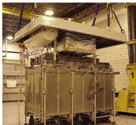
Fig. 2.29. Trial assembly of transformer coil assembly and top cover.
