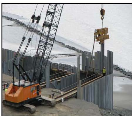
7a. Vibratory hammer driving the sheet pile.
