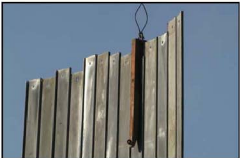
4. Hairpin weight used to set the sheet pile.
