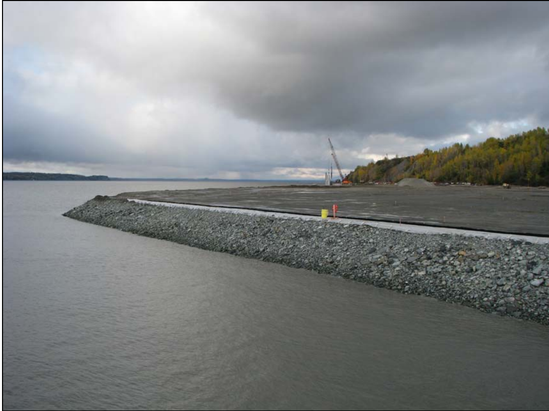
Figure 3(a). North Extension facing north.
