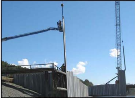
3b. Placing the sheet pile.
