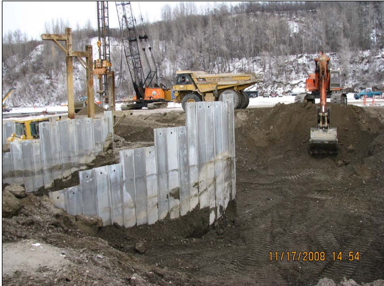
Figure 10. Out-of-water construction activities at barge berth site: constructing the tail walls of sheet-pile cells. View facing east.
