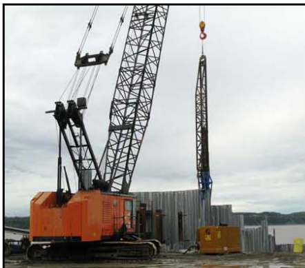
7b. Impact hammer driving sheet pile.
