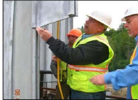
3c. Close-up of sheet pile being threaded.
