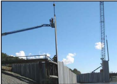
3b. Placing the sheet pile.
