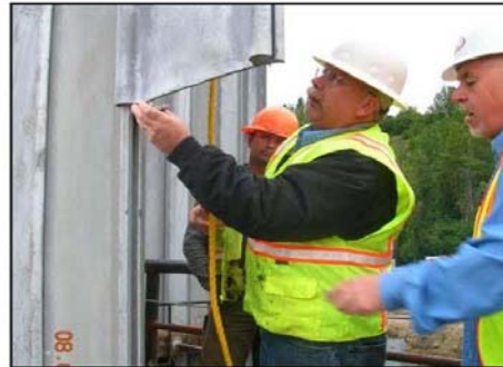
3c. Close-up of sheet pile being threaded.
