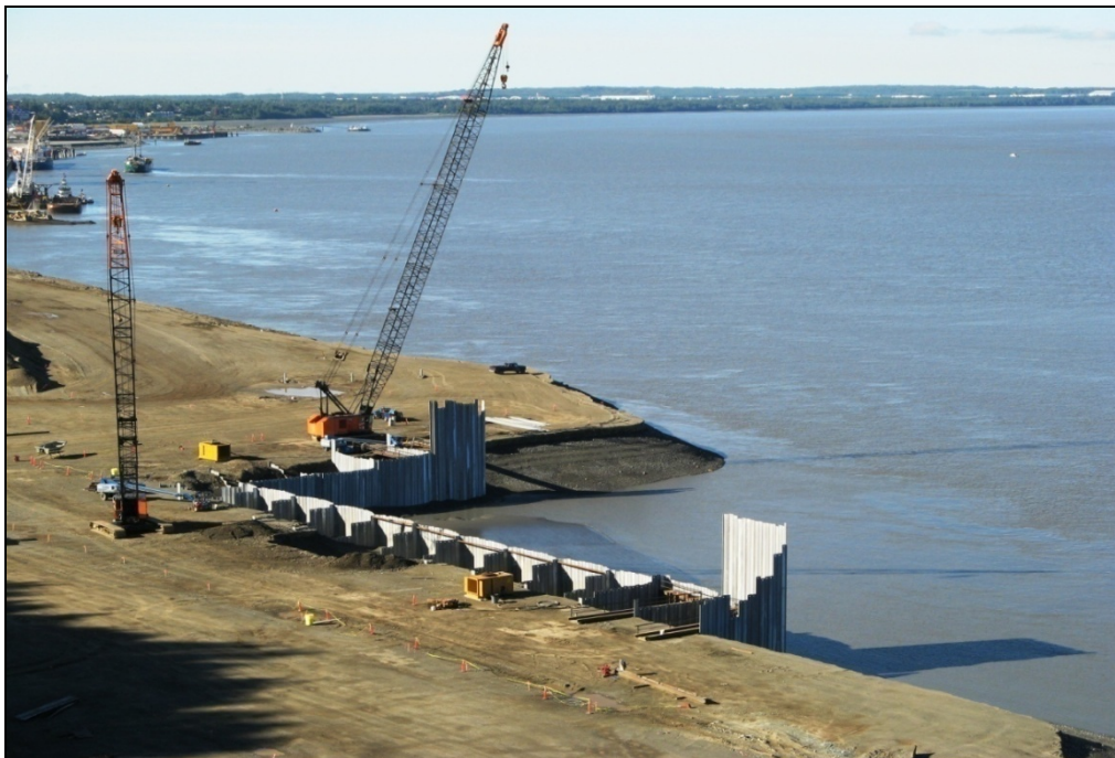
Figure 4(a). Barge Berth construction site, Port of Anchorage. August 2008.
