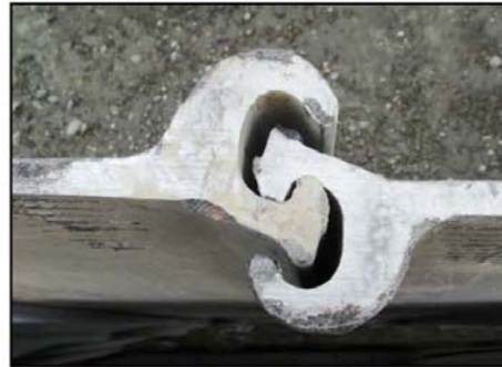
3e. Sheet pile "knuckles" interlocked.
