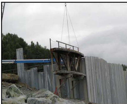
9. Template and soldier piles are moved to begin the next cell.
