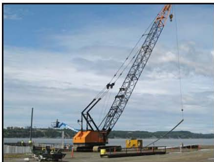
3a. Crane picking up sheet pile.
