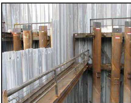
2. Walkway and template.
