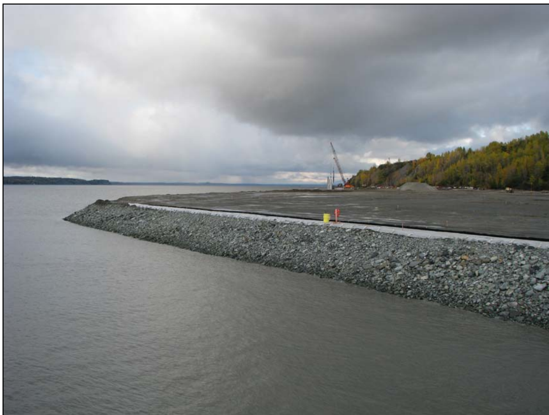
Figure 3(a). North Extension facing north.
