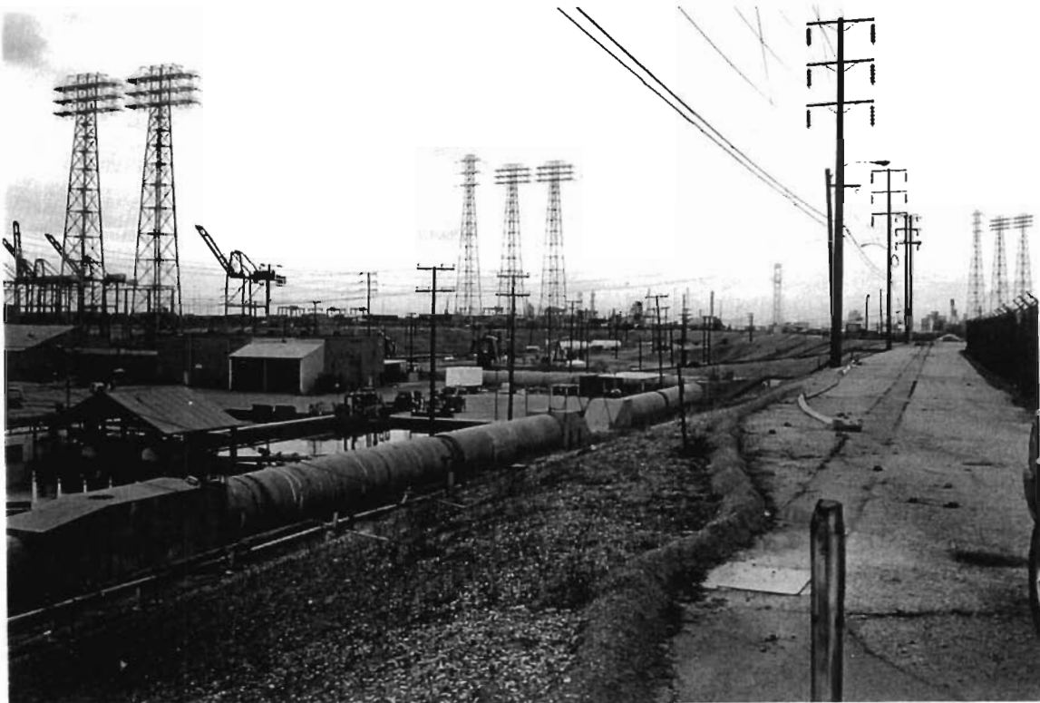
Photograph 4: View of onshore structures of Long Beach Generating Station.
