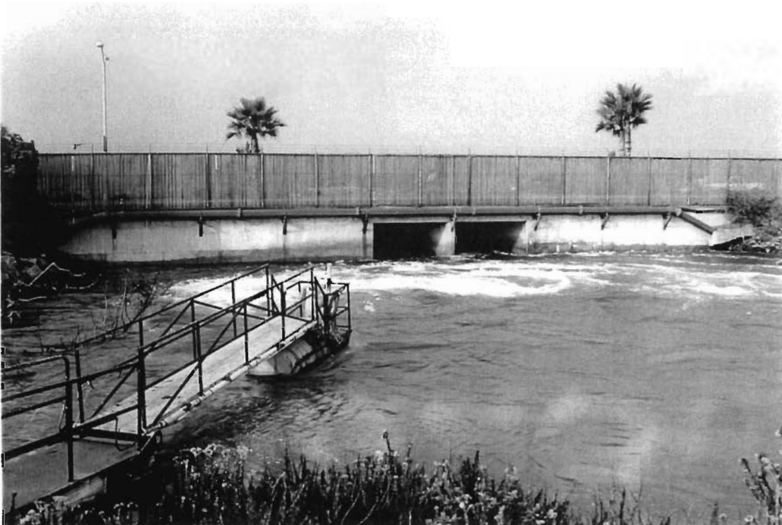
Photograph 4: View of outflow bay area.
