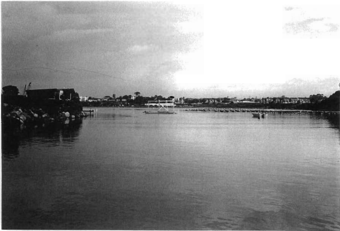
Photograph 1: View of Bay that leads to intake structure of the Encina Power Station.
