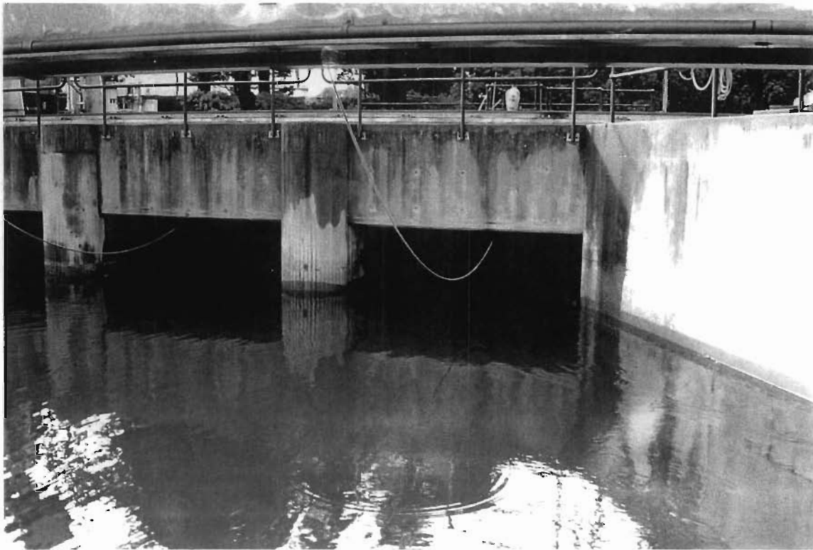
Photograph 2: View of intake structure; note low flow rate of the water.
