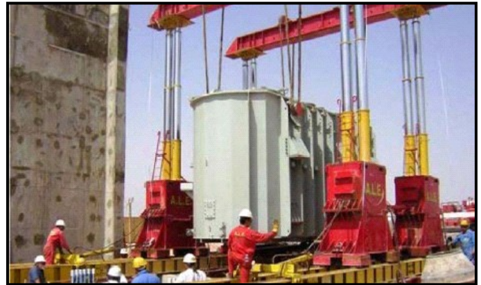
Placing a transformer at Kirkuk power plant
