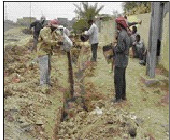
A Community Action Program water network reconstruction project.
