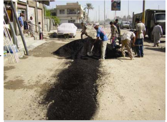
Paving over newly installed water mains
