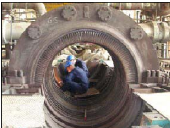
Work is progressing on the Unit 5 high pressure turbine
