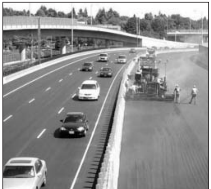
Figure 3 – Crews work without interruption on the I-84 (Banfield Freeway)
