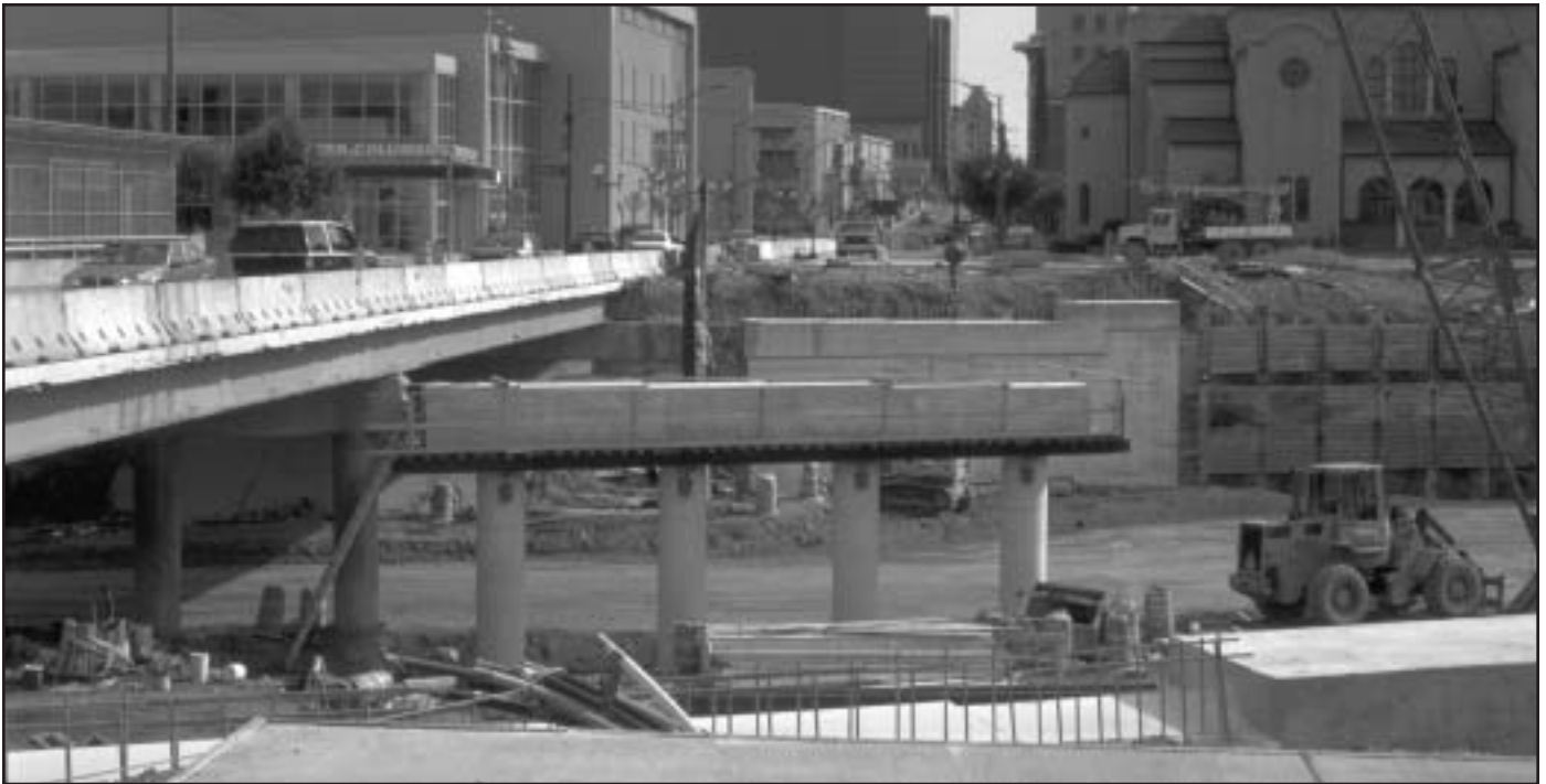
Figure 11 – Traffic crossing over the I-670 under full closure
