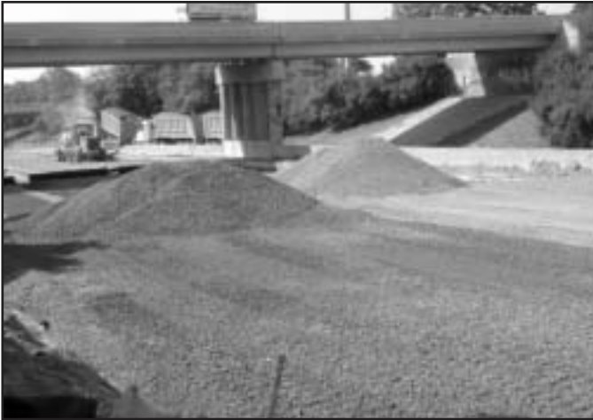
Figure 1 – Full closure increases available workspace for equipment and material
