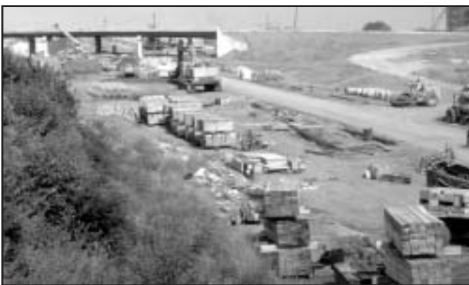
Figure 12 – Full closure increases available workspace for equipment and material
