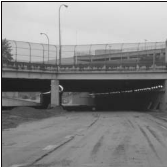
Figure 8 – The M-10 (Lodge Freeway) under full closure
