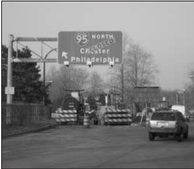
Figure 15 – I-95 North closed for construction
