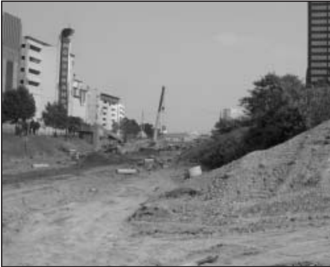
Figure 9 – Work being performed on the M-10 (Lodge Freeway) under full closure
