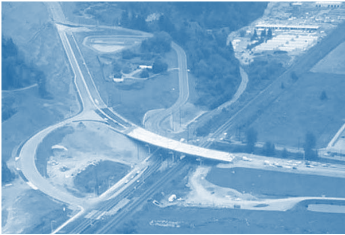
FAST Corridor project: New highway bridge over railroad near Tacoma. Source: FAST
