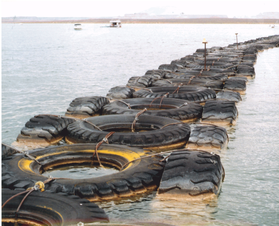
Tire breakwater - Glen Canyon National Recreation Area, Arizona.
