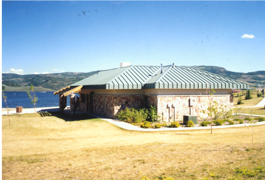
Comfort station and shower building - Jordanelle State Park, Utah.
