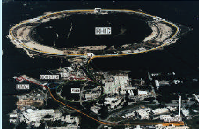
Figure III.B Aerial view of the Relativistic Heavy Ion Collider (RHIC) at Brookhaven National Laboratory. The beam from the Tandem van de Graaff travels to the Booster and Alternating Gradient Synchrotron (AGS) where it is accelerated further before being injected into the two counter-rotating rings at RHIC. In RHIC the beams are accelerated to very high energies (20 trillion electron volts in each beam for a gold nucleus) and then collided with one another. The RHIC accelerator and experiments are due to start operation in 1999.
