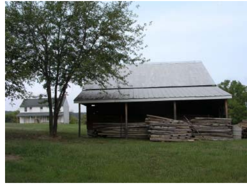
NPS recently restored historic buildings damaged during a storm at the Lewis Farm on Monocacy National Battlefield in Maryland.
