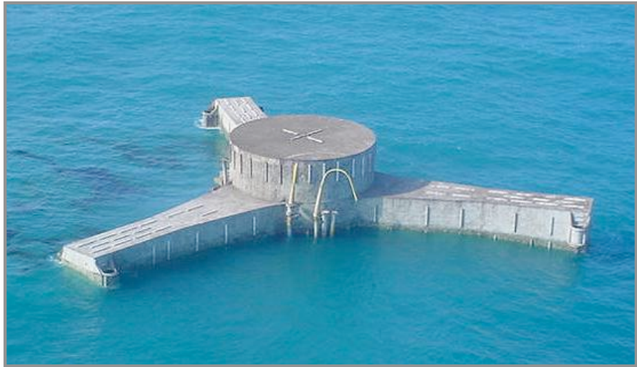
Figures 3.4a and 3.4b. Hurricane damage at the Mars drilling platform in the Gulf of Mexico – Typhoon platform
