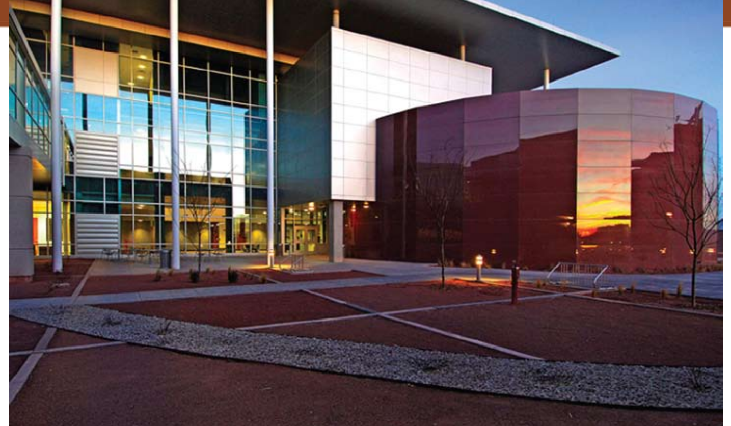
The setting sun reflects off the glass of the cylindrical training center attached to Sandia's new MicroLab building, the second of three to come online of $500 M MESA project. (Photo by Bill Doty)
