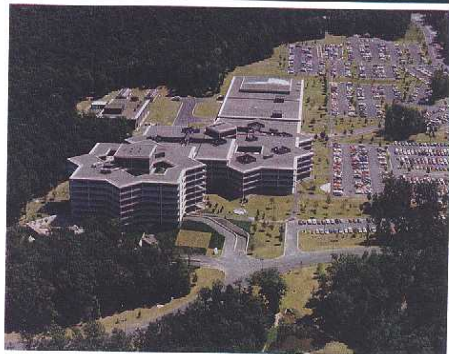
The John Wesley Powell Building, Reston, Virginia (taken 1978). Seven stories of unfaced Portland cement and glass comprise nearly 1 million ft 2 of office and laboratory space. Courtesy of the U.S. Geological Survey.
