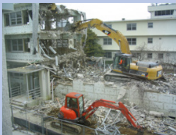
Caption: Demolition on Building E-108.
