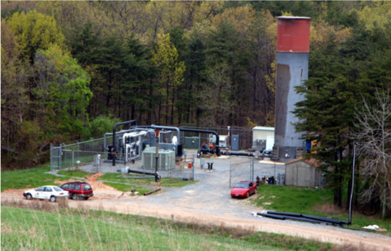
Caption: Landfill Gas Processing Plant, Sandy Hill Landfill. This plant purifies the gas before sending it to Goddard Space Flight Center.
