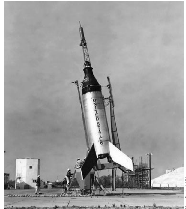
Crews prepare a Little Joe rocket for launch from Wallops Island. The Little Joe project tested escape systems for the Mercury capsule and biomedical conditions during rocket flight in the early 1960s.
