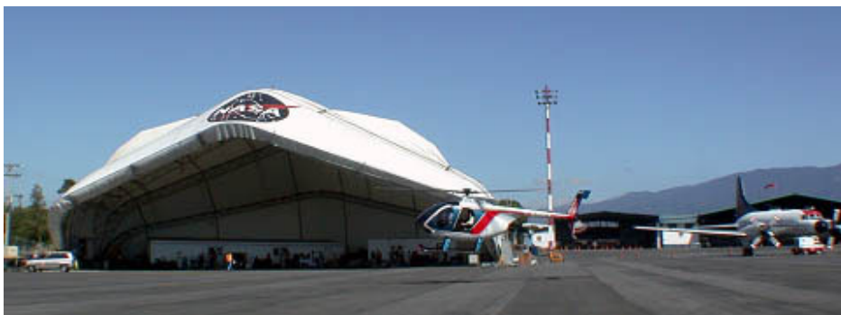
The Pre-AVE mission was staged from the Costa Rica National hangar of Aerotransport Investigations (Hangar Nacional de Investigaciones Aerotransportadas, Juan Santamaría, Costa Rica) also known as the clam-shell hangar.
