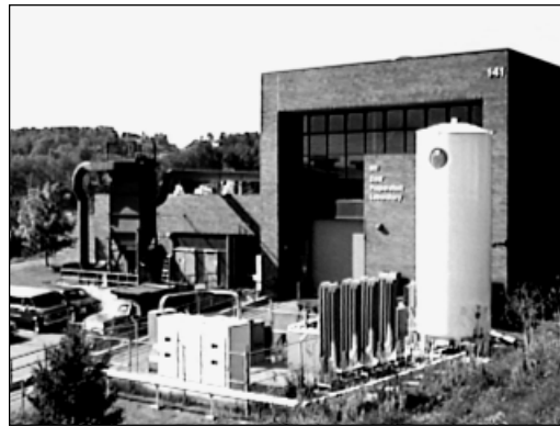
FETC's Solids Processing Research Facility is a fully integrated, 100-2,500 lb/hr continuous bench-scale facility for testing innovative, emerging solids processing equipment and technologies.
