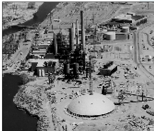
Aerial view of Piñon Pine IGCC with raw coal storage dome in foreground and the gasification and power island in background.
