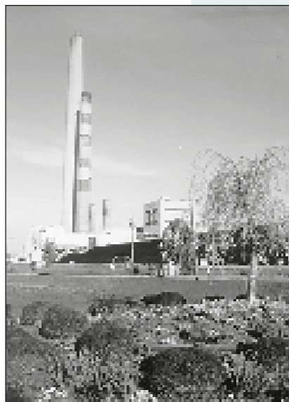
GNOCIS was developed at Georgia Power Company's Plant Hammond to optimize the low-NO x techniques developed in the CCT Program.
