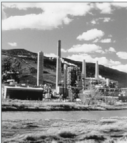
Sierra Pacific will demonstrate an air-blown, fluidized-bed gasifier with hot gas clean up at the Piñon Pine CCT project.
