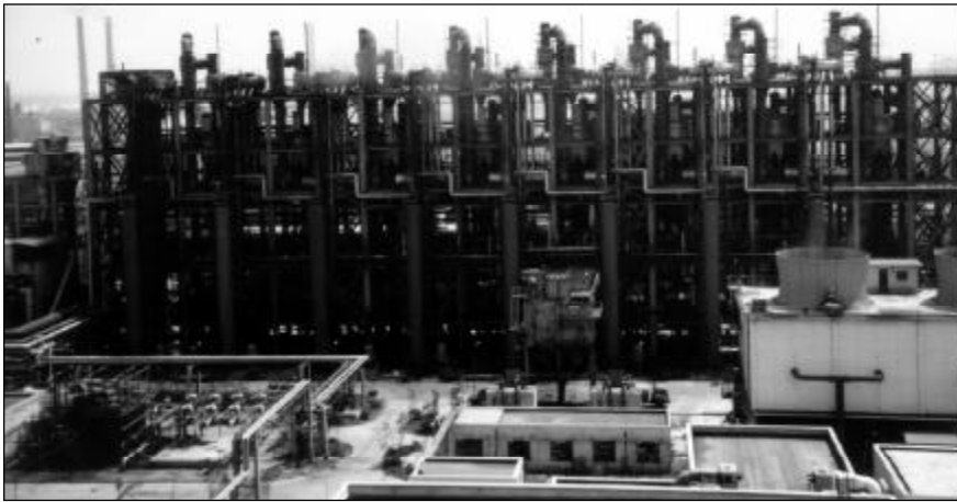
The Shanghai U-GAS Gasification plant, in operation since 1994
