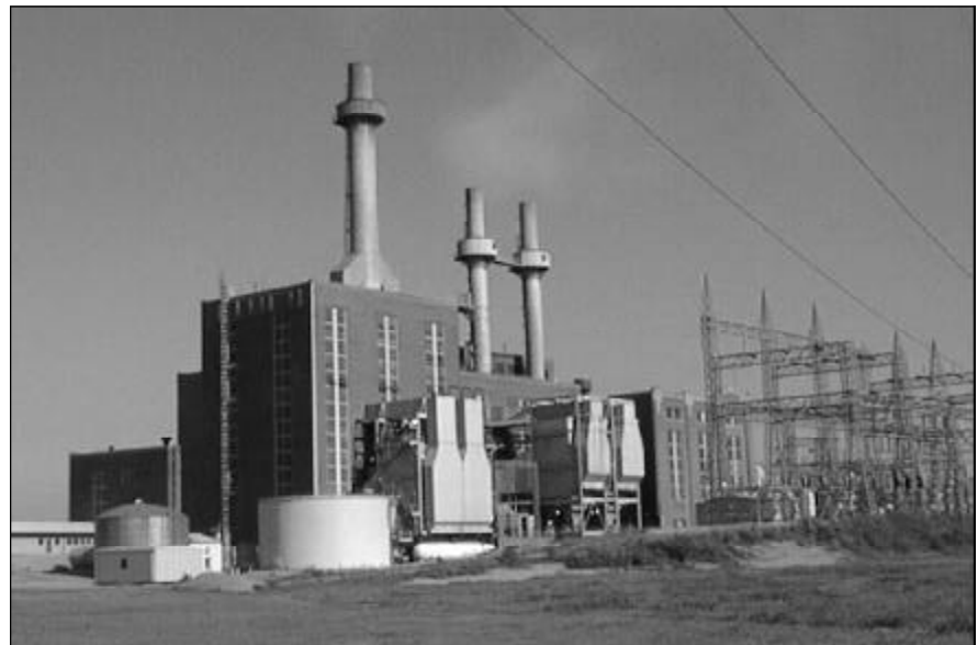
Southeast view of the 186-MW Grand Tower Plant
