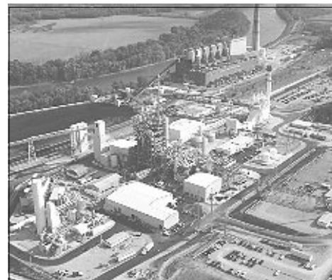
All major equipment, including the gasifiers, air separation unit, and gas turbine, has been installed in the Wabash River Plant. The plant became operational on December 1, 1995
