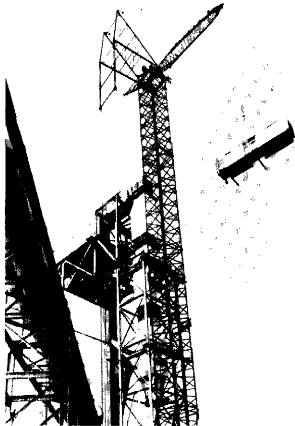
Large section of new flue gas bypass duct being lifted into place by tower crane onto existing FGD duct.
