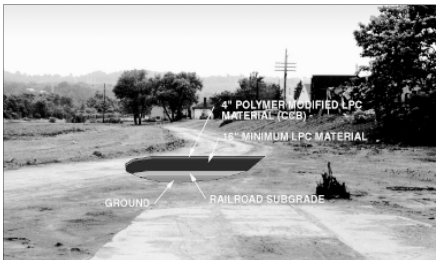
Figure 3: "Rails to trails" demonstration project using CCB materials
