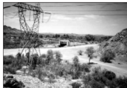
In the Tubac, Arizona project, new transmission line would parallel existing lines
