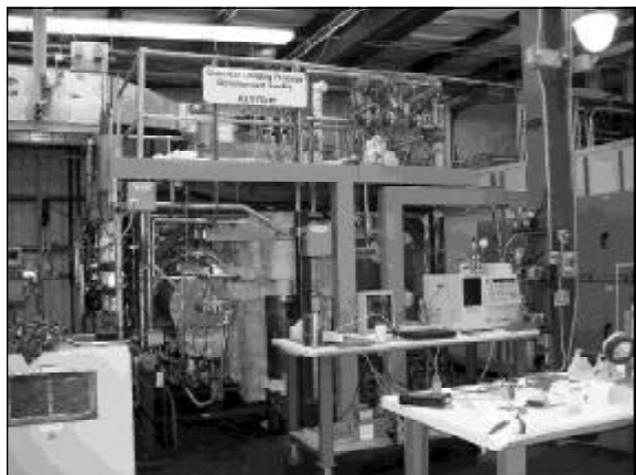
Alstom's Chemical Looping Gasification Process Development Unit in Windsor, Connecticut
