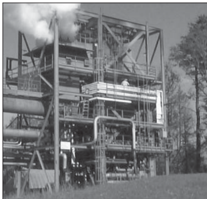
Alstom Power Inc.'s Boiler Simulation Facility
