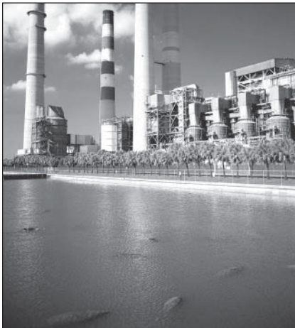
Tampa Electric's Big Bend station has four pulverized coal electric generating units. The project is to apply the NN-ISB system to Unit #2, a 445-MW wet bottom unit firing high-sulfur eastern bituminous coal
