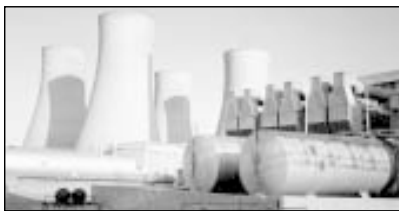
Komati Power Station's cooling towers and electrostatic precipitators
