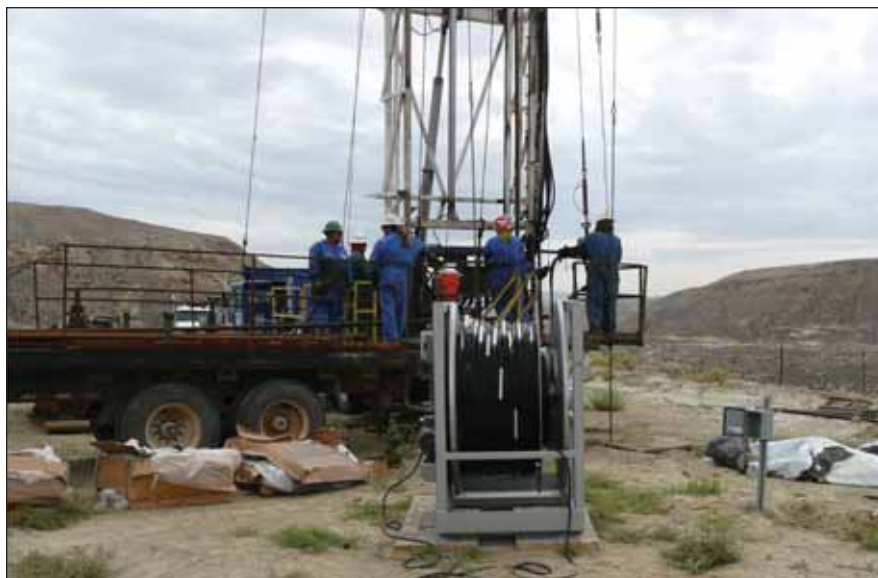
Installation of seismic geophones at SWP’s Aneth Phase II project
