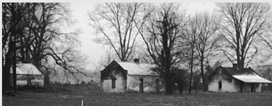
Quarters at Cane River Creole National Historical Park. Photo by the author.
