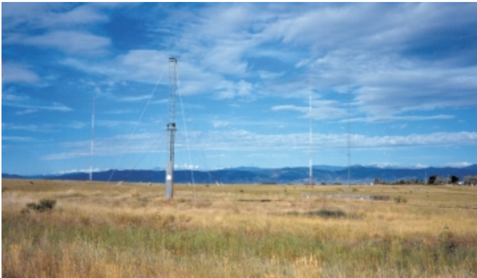
Figure 3.4. 15 MHz WWV Antenna (WWVB Towers in Background)
