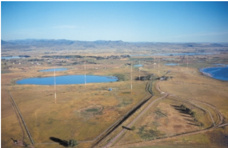
Figure 2.1. Aerial View of WWVB/WWV Station Site
