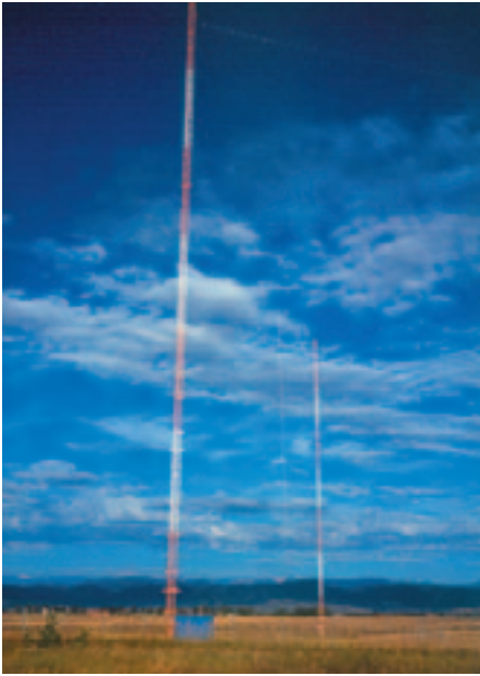
Figure 2.2. WWVB Antenna Towers
