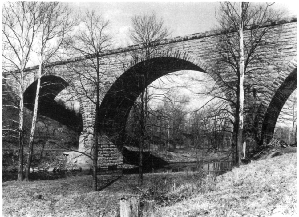
The Baltimore and Ohio Viaduct over the Black River, near Lodi, Medina County, Ohio, is a monumental masonry civil engineering structure. The photograph shows the timeless simplicity of the stone arched viaduct built in 1892 on the main line of the Baltimore and Ohio, linking Chicago with the East. (Eric Johannesen, 1975)
