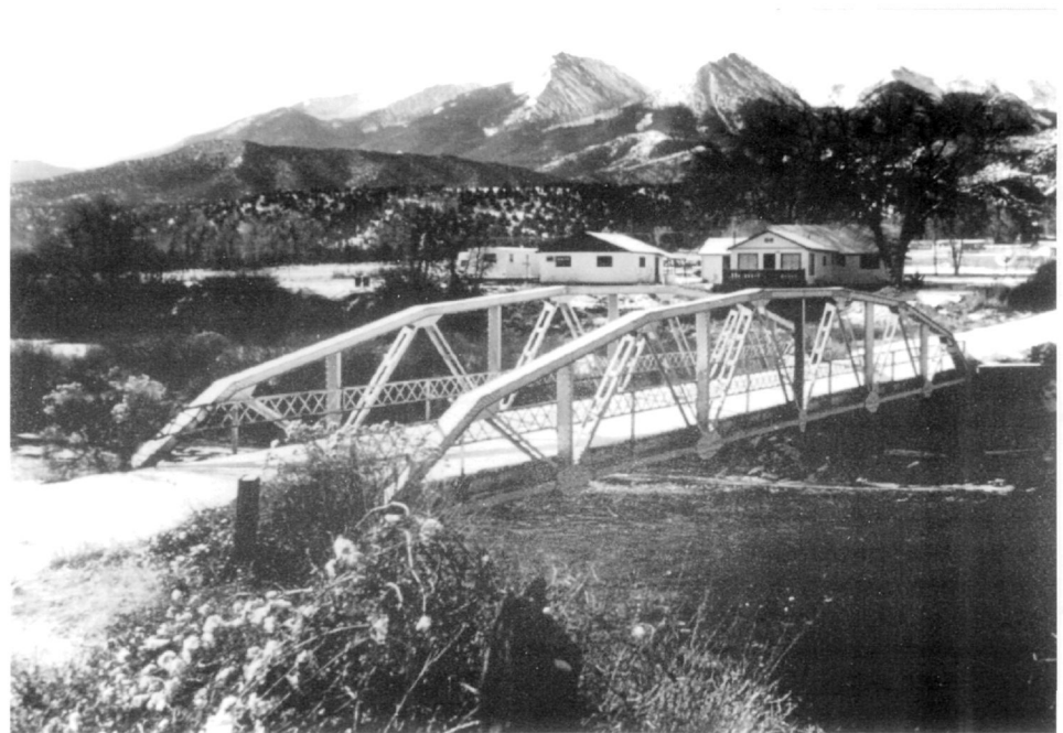
View from the Northeast of the Howard Bridge in Colorado, showing the structure and approaches to the bridge. (Clayton B. Fraser, 1983)
