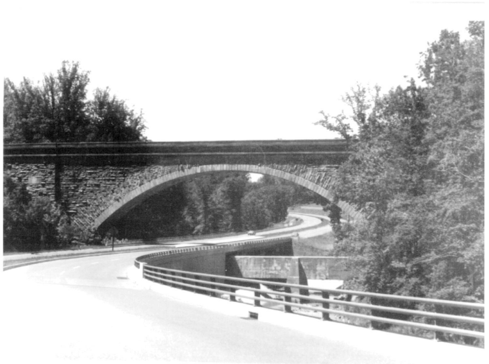
Cabin John Aqueduct, Montgomery County, Maryland. This stone arch was built in 1869 and was the world's longest until 1903. It was designed by Montgomery Meigs, U.S. Army Corps of Engineers. The aqueduct provided the principal source of water to Washington, D.C. throughout the late 19th century. (Michael Bourne, 1969)
