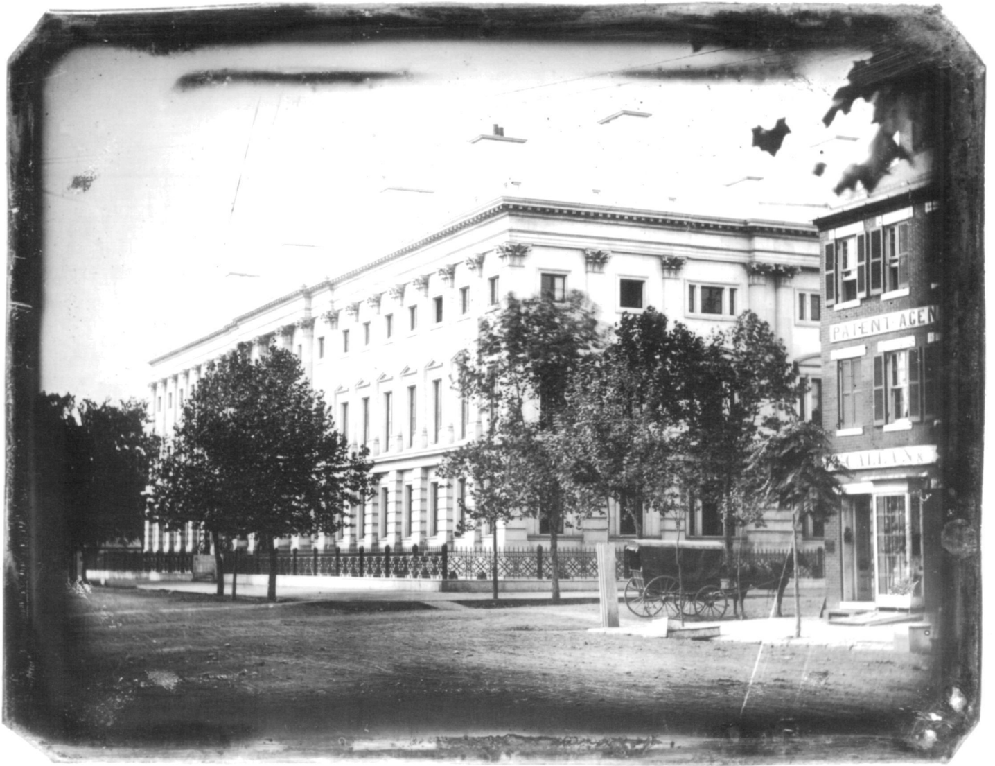
The General Post Office, Washington, D.C., 1839, designed by architect Robert Mills. This photo is a copy of a daguerreotype of the building taken in 1846 by John Plumbe. (Library of Congress Daguerreotype Collection)
