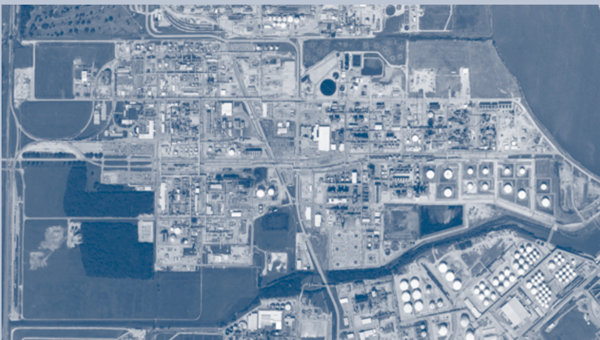
Rohm and Haas plant in Deer Park, Texas
