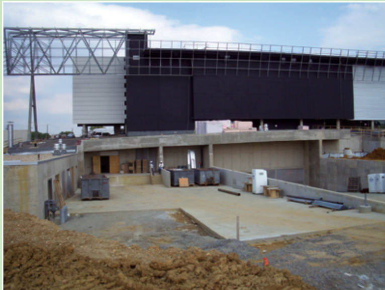
Construction of the NOAA Satellite Operations Facility in Suitland, MD.
