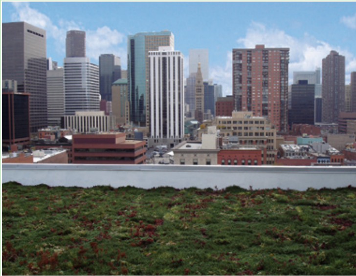
In addition to the solar park, the Federal Center in Denver, CO also has a green roof.
