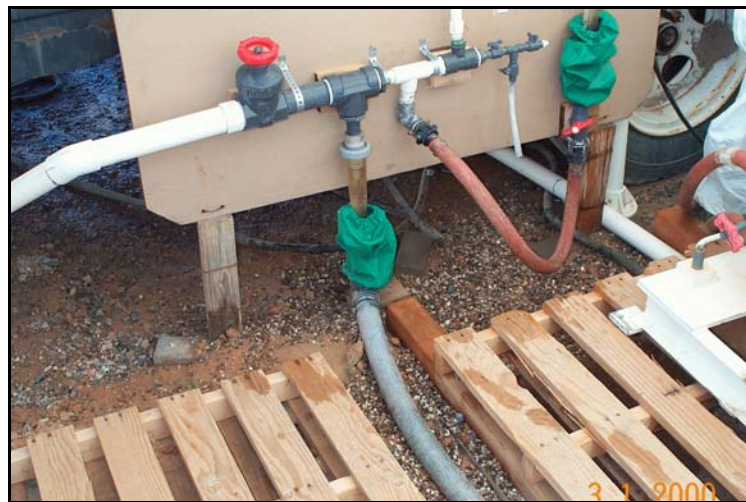
Figure 6.—SSF outlet flow control structure.
