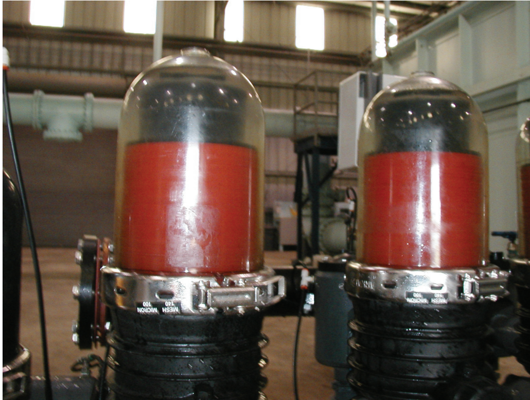
Figure 5.1 Close-up photograph of disc pre-filtration technology, supplied by Arkal/ A2 Water.
