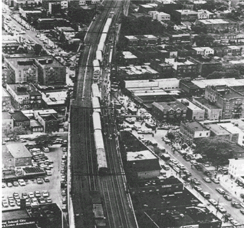
Figure 5. Incident with sawtooth lateral buckling; New York, New York – July 23, 1984
