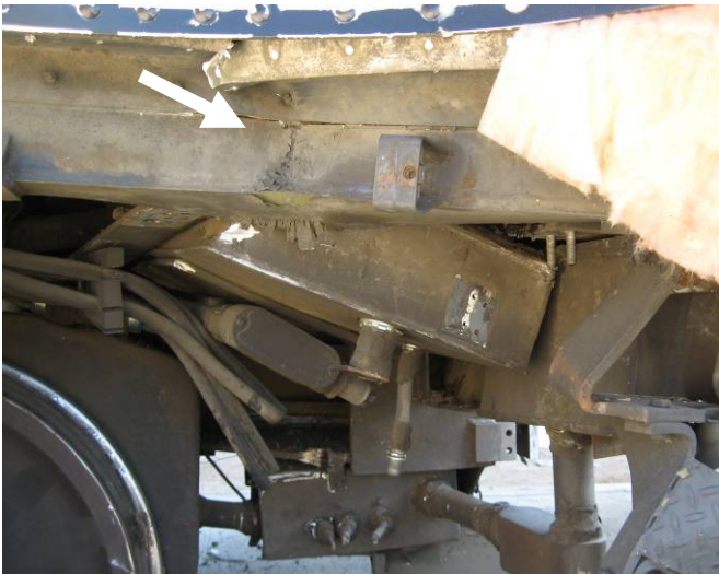
Figure 16. Lateral Buckle of the Right Side Sill
