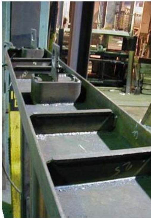
Figure 25. SOA End Frame in Fabrication; This is the AT plate Before the Top Plate was Welded on
