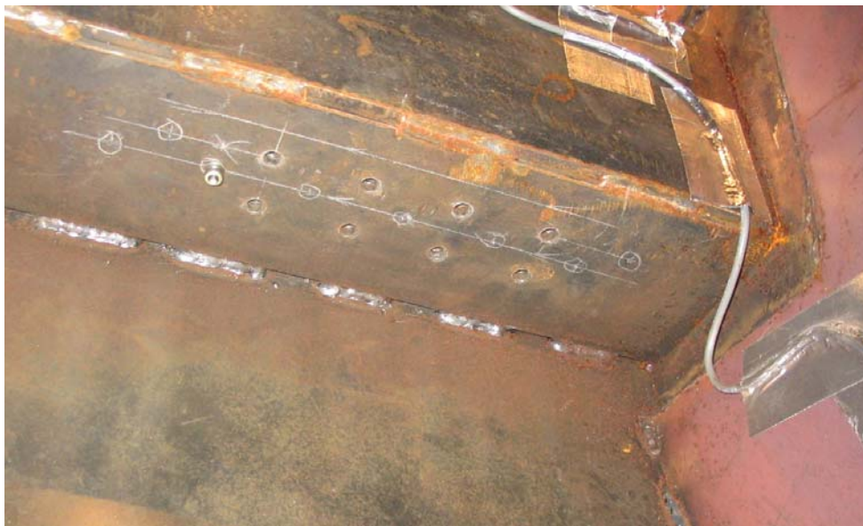
Figure 28. Rivet Pattern for the Repaired Roof Absorber Shear Joint (Bottom Surface)
