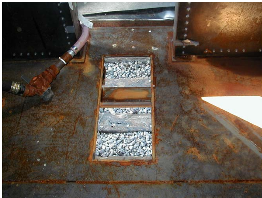
Figure 15. Access Hole Cut in the Floor Plate in the Vicinity of the Sliding Sill/Fixed Sill Connection
