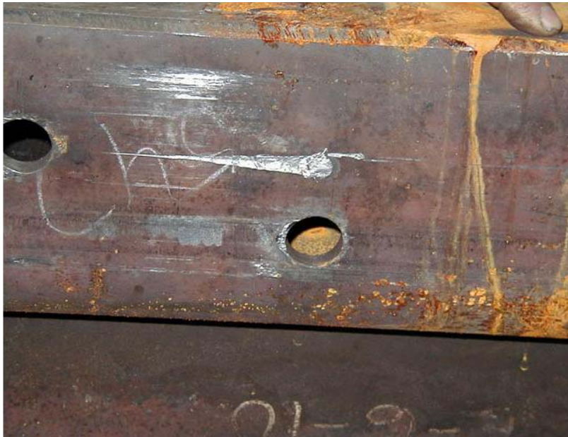
Figure 5. Bolt Hole in the Sliding Sill of One of the Crush Zones After the Test
