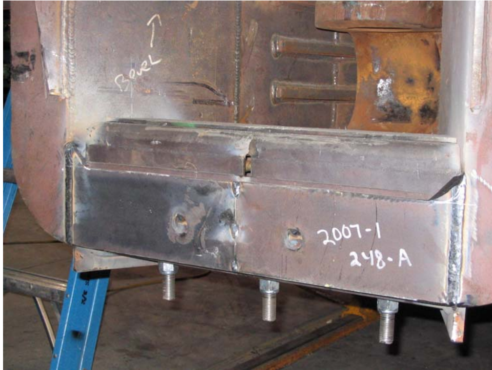
Figure 16. Bell-Mouth Face Plate Repair
