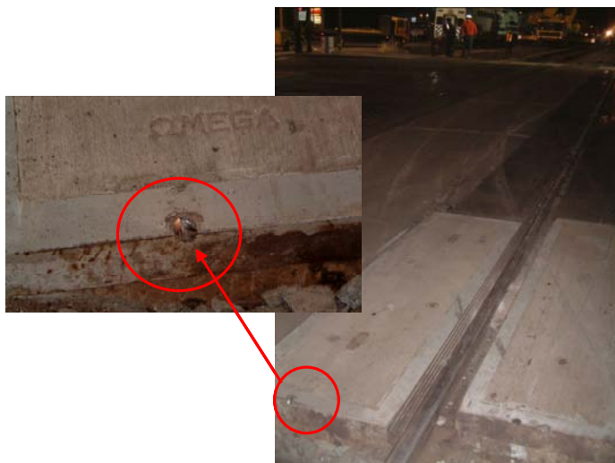
Figure 16. Site Photograph of Concrete Embankment at Highway-Rail Grade Crossing
