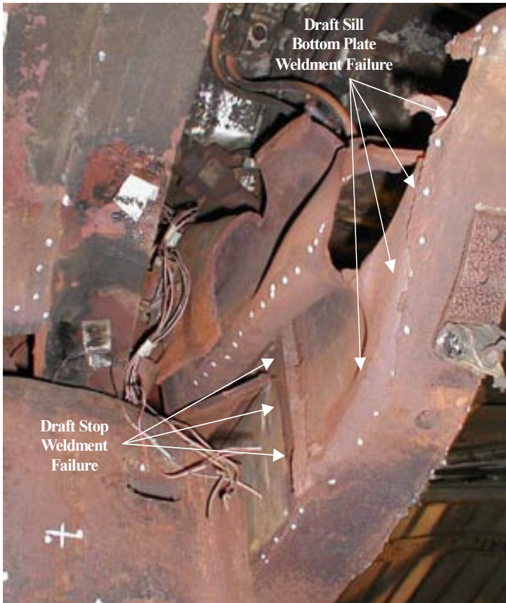
(a) observed draft sill weldment fractures
