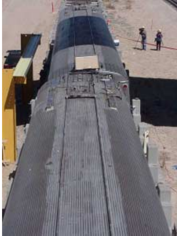
Figure 6-7. Photo of Coupled Connection After Two-Car Test
