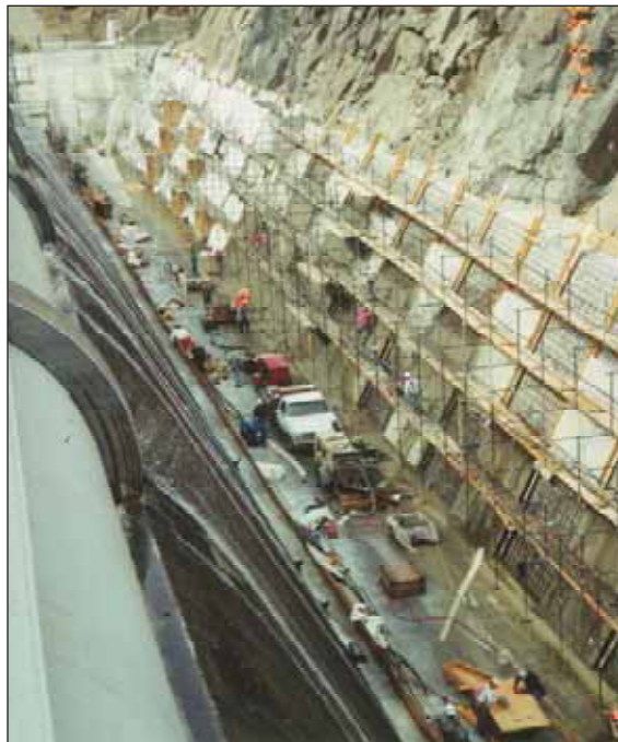
3.8. Tieton Dam spillway rehabilitated in 1999.
