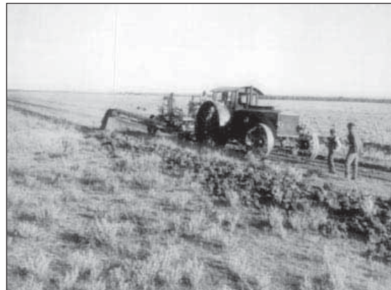
4.1. In October 1913 a Pioneer traction engine pulled an Austin elevating grader digging drainage ditches on the Milk River Project near Malta, Montana.
