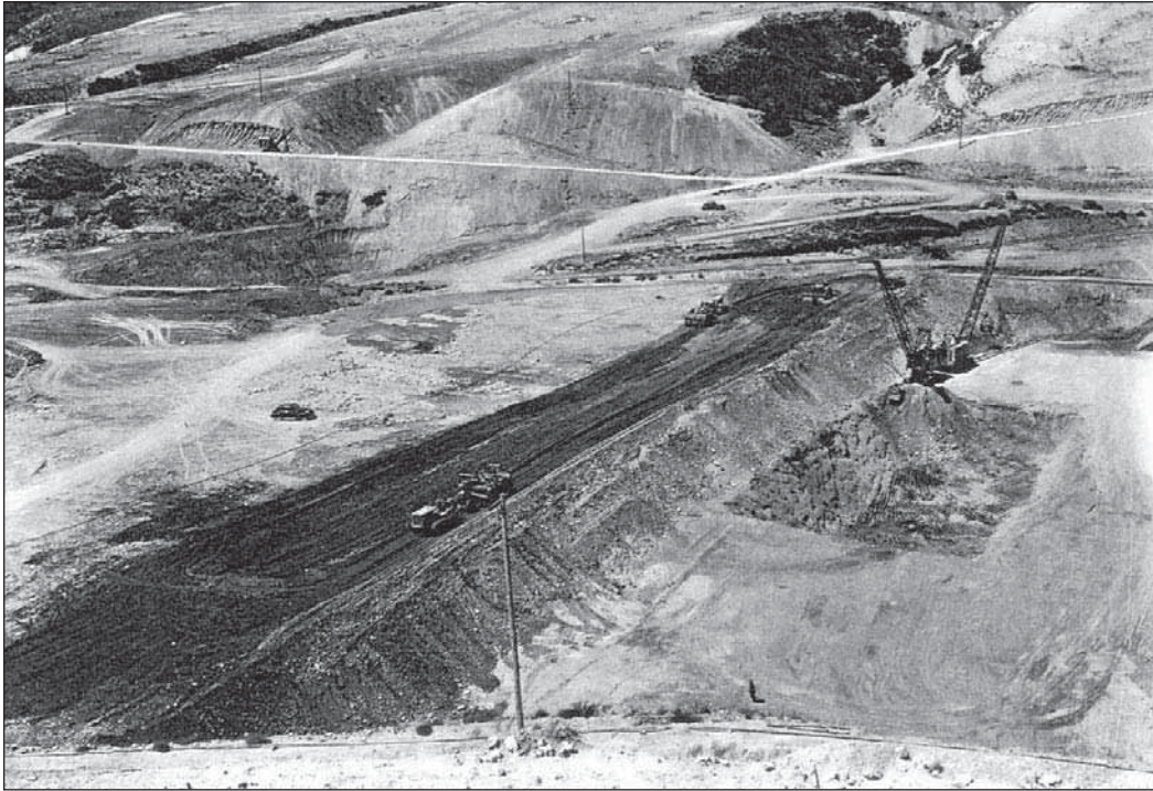
17.4. Construction at Deer Creek Dam.
