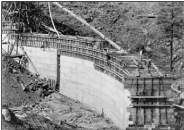
1.13. Construction of Gerber Dam. Note closure slot near left side of photo.
