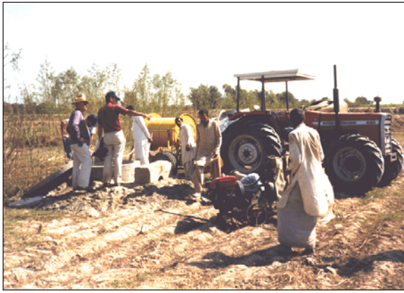
28.4. Reclamation advisors assist Pakistani counterparts in drainage work.
