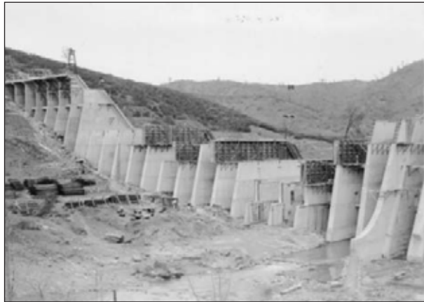
1.14. Photo taken during construction of Stony Gorge Dam, California from downstream side. Note struts between buttresses and sloping slabs on left side of photo.
