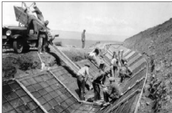
3.5. Delivery of concrete by truck from a centrally located concrete plant.
