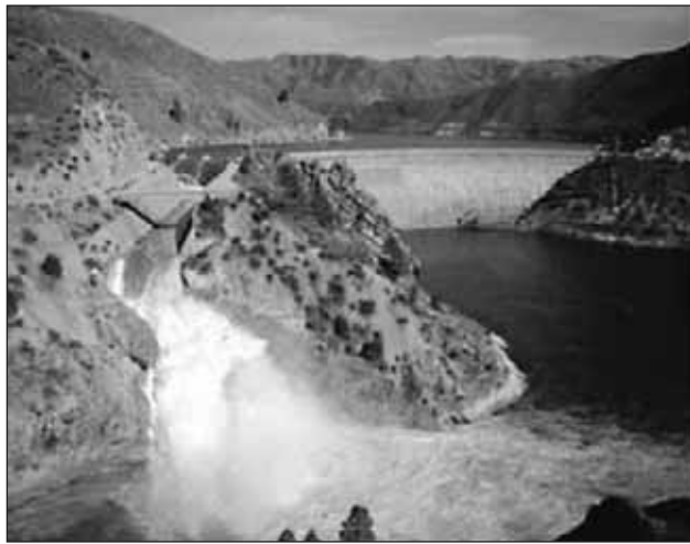
1.8. Arrowrock Dam, Idaho.
