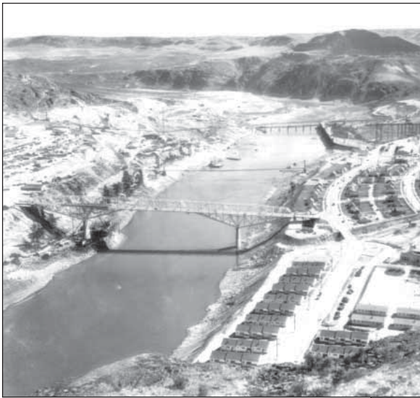
35.1. Grand Coulee Dam construction in 1936.
