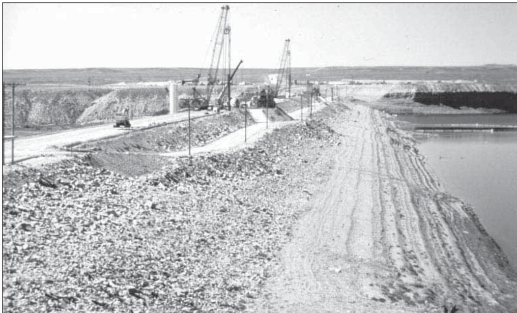
2.19. Fontenelle Dam: Diaphragm wall construction.
