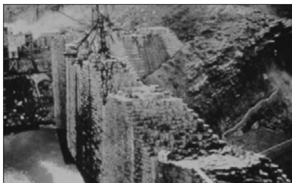
1.3. Masonry Construction at Theodore Roosevelt Dam, Arizona
