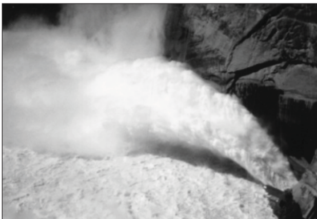
1.29. Basin X (tunnel flip bucket), spillway discharging approximately 27,000 ft 3 /s - Glen Canyon Dam, Arizona.
