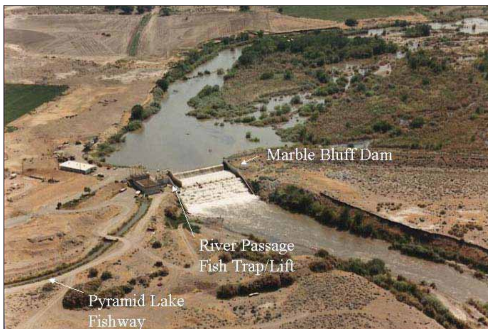
6.5. View of Marble Bluff Dam and the exit of Pyramid Lake Fishway.
