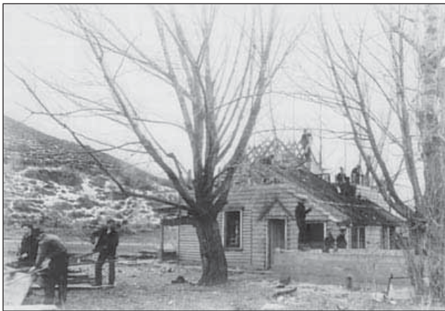
17.3. This 1940 photograph by Ellis Armstrong, later a Commissioner of Reclamation, shows CCC forces dismantling the Atwood house in the Deer Creek Reservoir area near Charleston on the Provo River Project.
