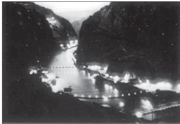
18.1. Black Canyon during early preparations for construction of Boulder Dam.
