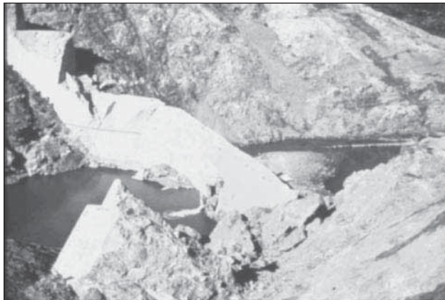
1.40. Malpasset Dam failure, Cannes District, France.
