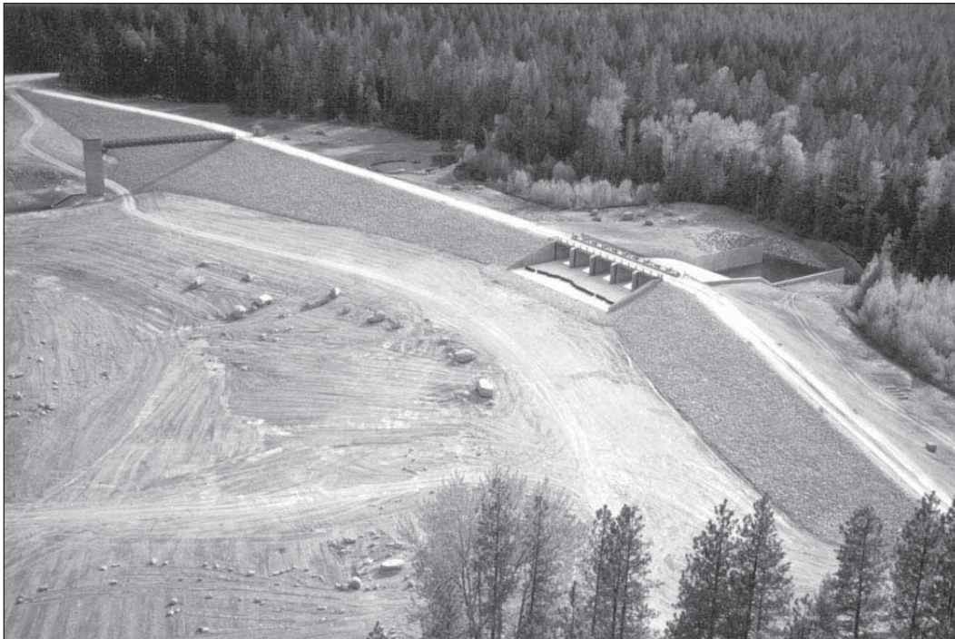
2.22. McDonald Dam: New dam in 2000.
