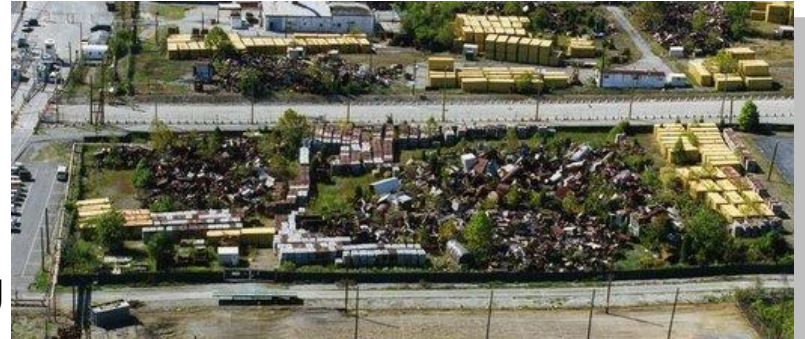
This old scrap yard at Y-12 will be one of the first cleanup projects to be done with stimulus money in Oak Ridge.
